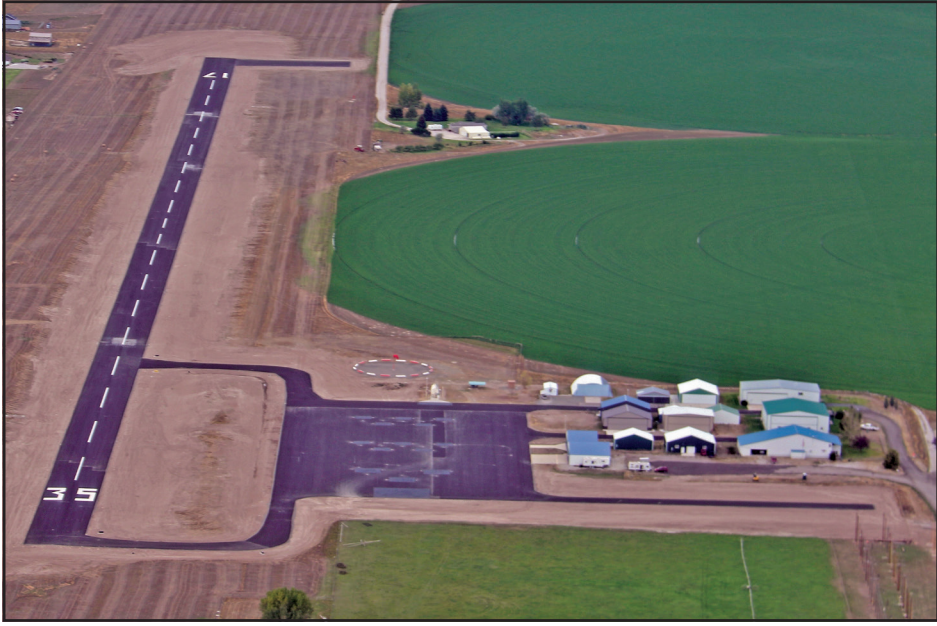
Broadwater County Airport is now open for flight operations. Photo Credit: Matt Nelson
