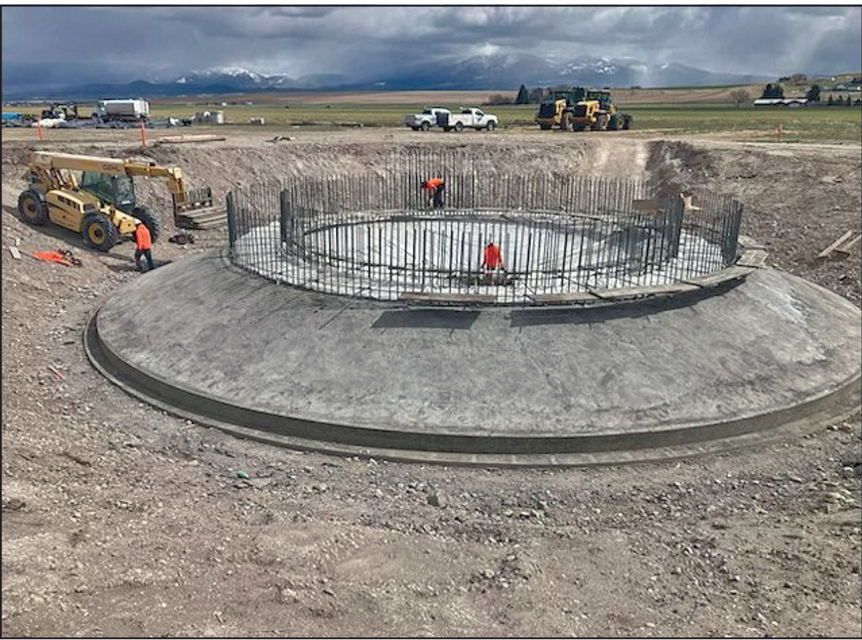
COPs Construction crews have poured 450 cubic yards of concrete for the massive footing. The footprint of the site is one acre, part of the 76 acres the City owns at the corner of Highways 12 and 284.
