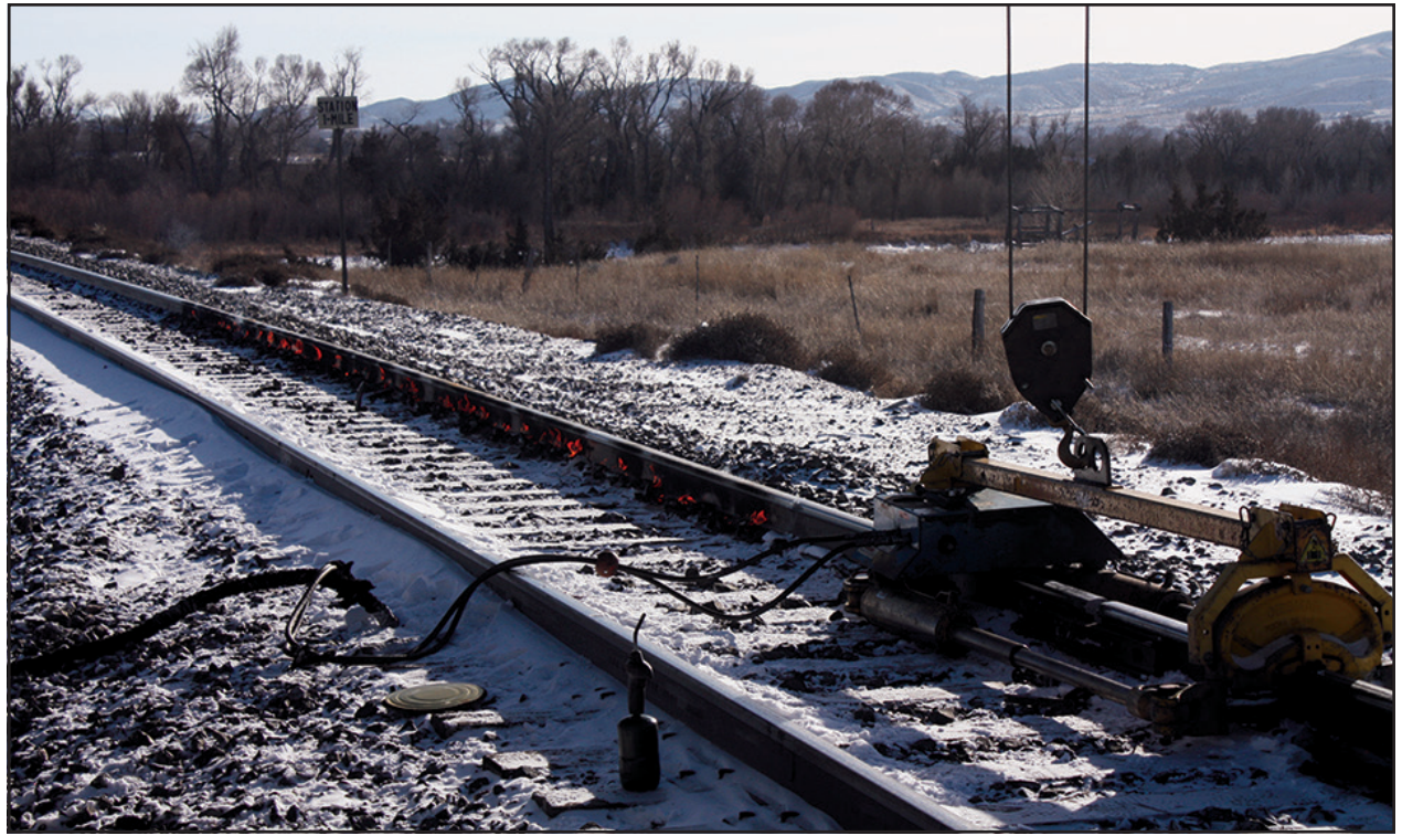
Railroad maintenance crews were tasked with heating steel rails with blow torch fires to reconnect rail sections that had separated on Saturday Photo Credits: Nancy Marks
