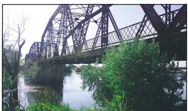
Bridge at Toston, Montana. Photo Credits: Nancy Marks
