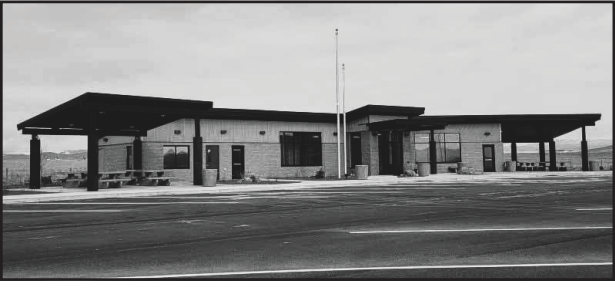
New Rest Area on Hwy 287 at Wheatland Photo Credit: Nancy Marks
