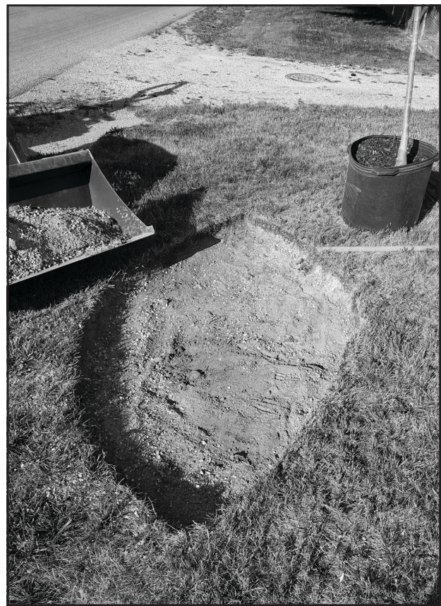
Eye-shaped bed after sod-removal and excavation to 3-4 inches deep. Photo Credit: Pat Plantenberg
