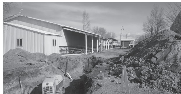
Waste Water Work Under Way
