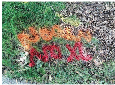
Locate service has marked this property indicating there is no Electric (red) or telecommunication lines (orange) in the area.
