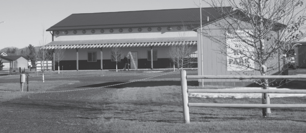
Carpenter building awning on new building Three Forks Market RV Park and Campground.
