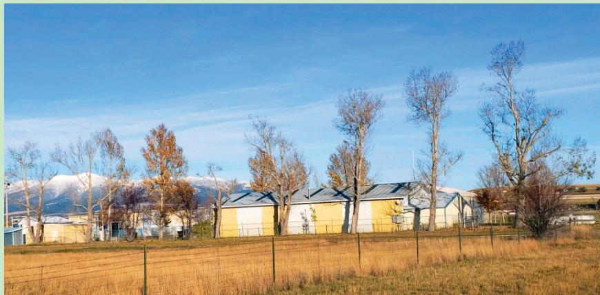
Seven of the eight large hazard trees removed at the Fairgrounds west of the 4H Building (Photo by Pat Plantenberg)
