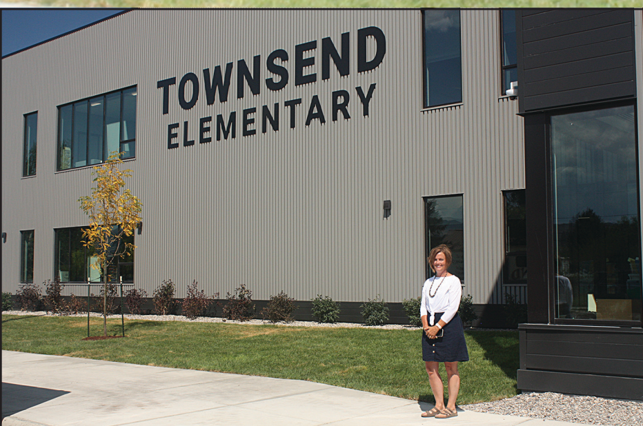
Townsend Elementary School Principal Christina Hartmann proudly displays the front of the new grade school.
